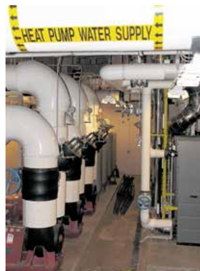
Submitted Some of the pumps for the geothermal system at Great River Medical Center in West Burlington, Iowa.
